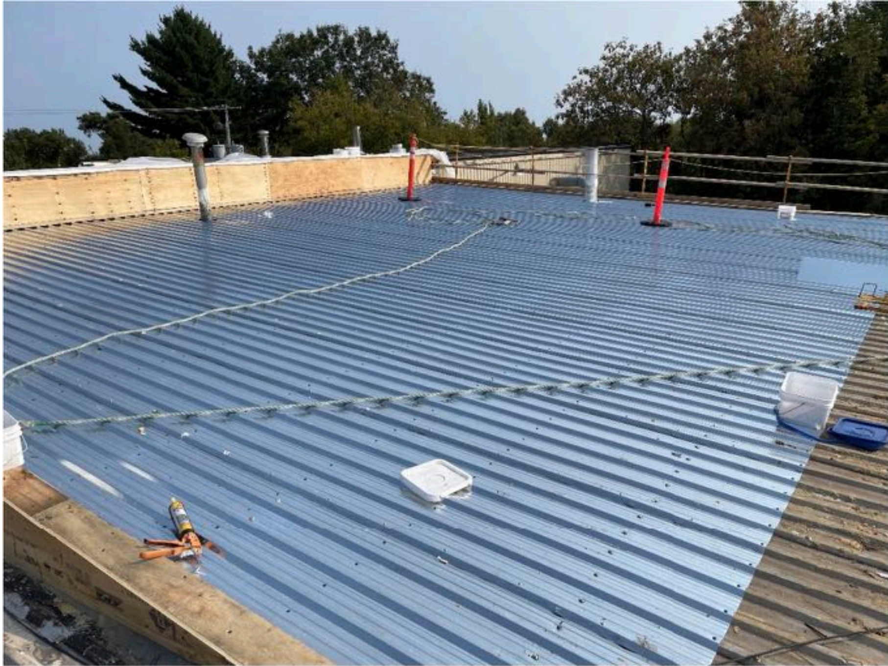
5.2 New Roof Panel Installation Complete
