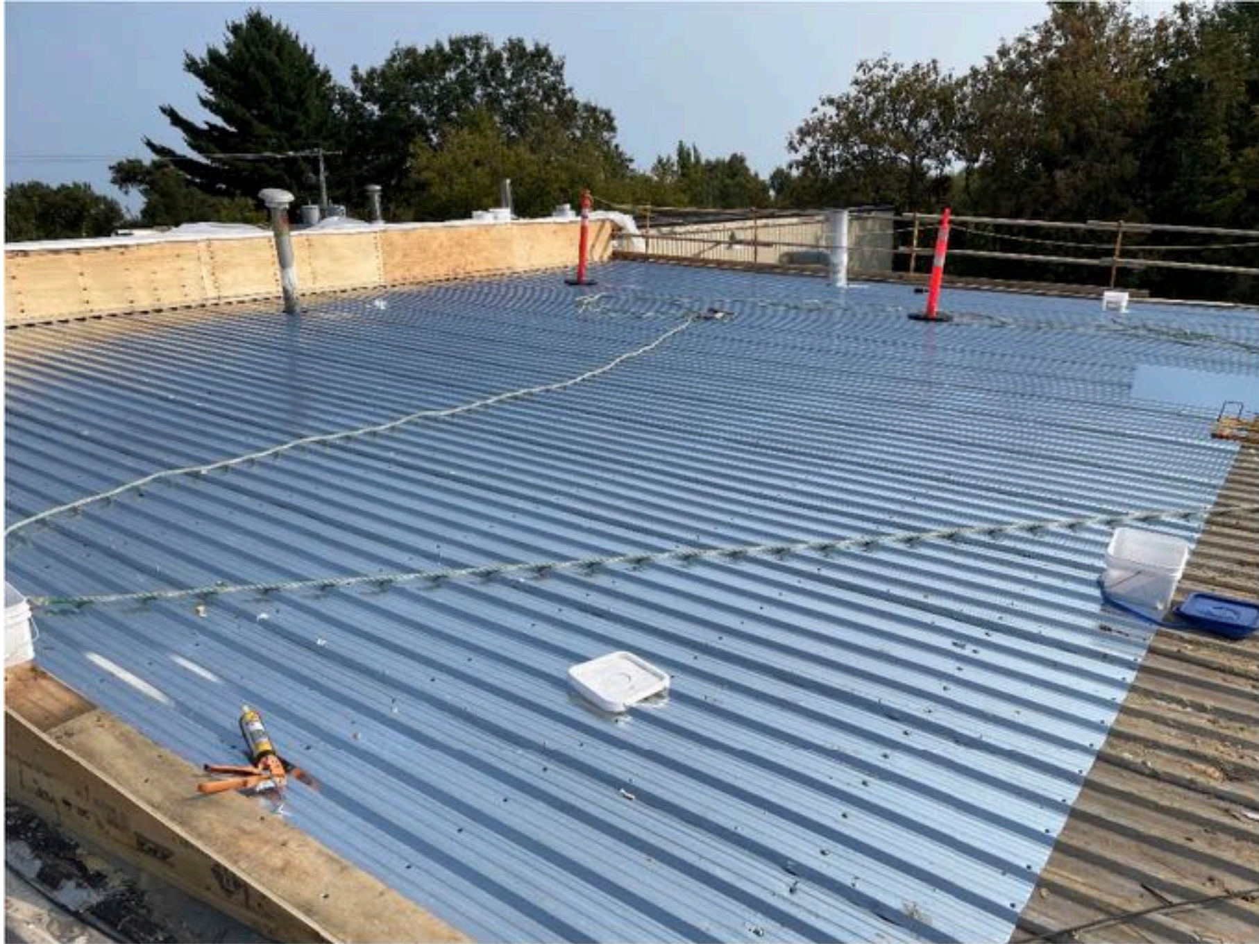
5.2 New Roof Panel Installation Complete
